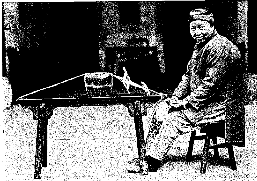
FIG. 268. RIBBON LOOM.
