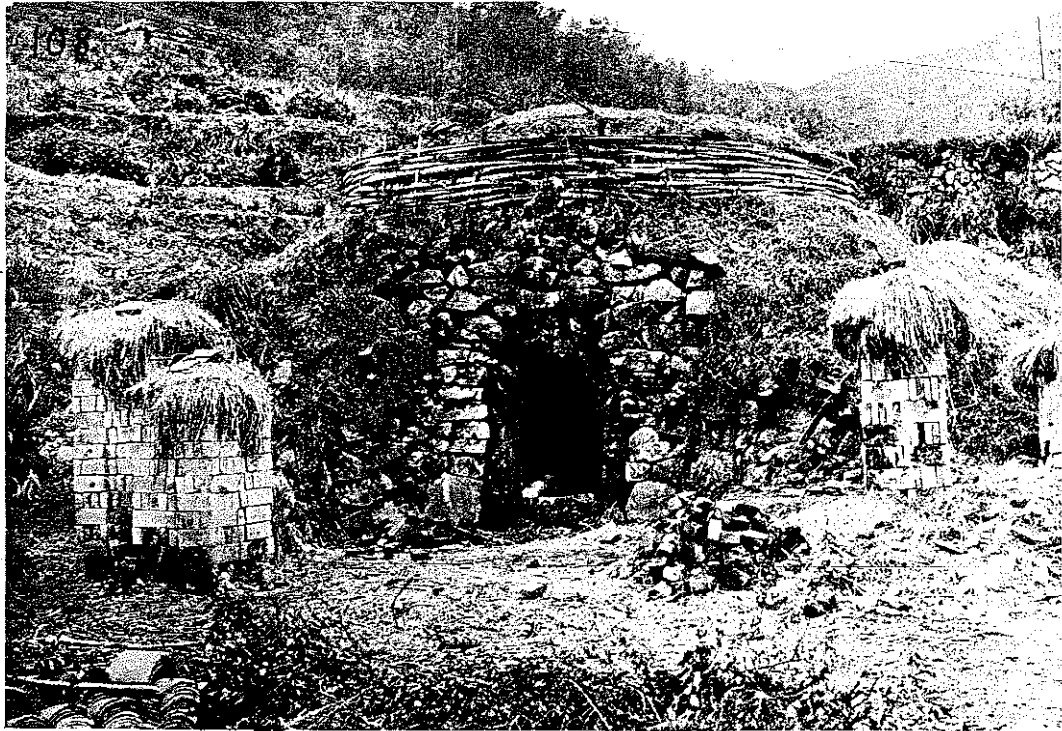
FIG. 392. KILN FOR BURNING BRICKS AND ROOFING TILES.
