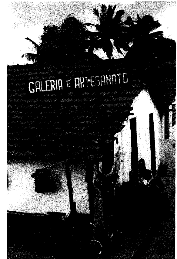
Abb. 3.11 Tonziegeldach in Brasilien Fig. 3.11 Clay tile roof in Brazil
