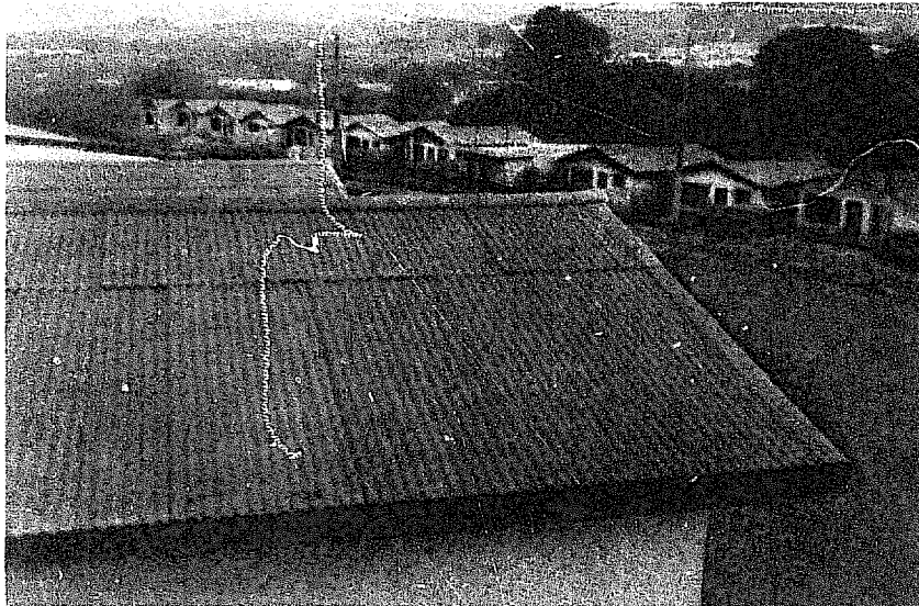
Fig. 5.15 Asbestos cement roof.
