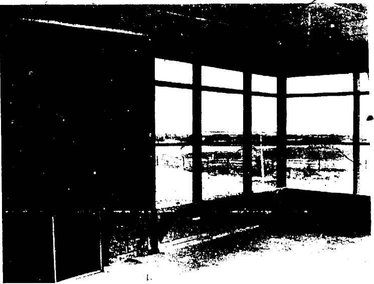
LIVING ROOM CORNER faces southeast and has floor-to-ceiling fenestration of simple design. There is no sash in conventional sense. Both the louvered ventilation panels and the glass itself are set directly in a dressed 2 x 6 in. frame. Where it abuts earth walls, this frame is bolted into a groove formed to receive it.
