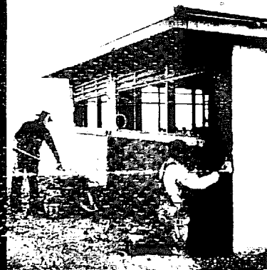
EXTERIOR SURFACING on Miller house consists of dagga-cement plaster, brush-finished with water-proofing and finished with a cement base paint. Local failures in this finish led to tests of new formulae.
