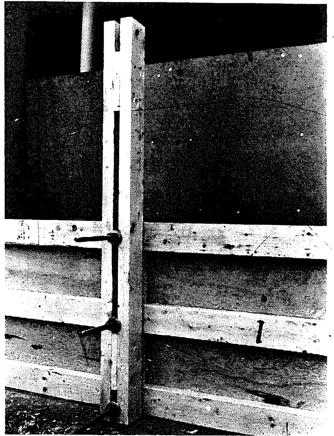
Close up view of panels 1, 2, 3.
