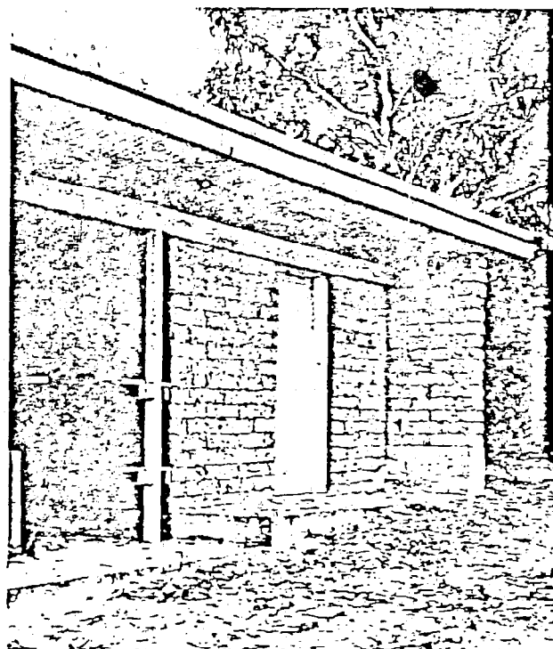
Experimental pavilion of unrendered adobe blocks 20 years after construction
