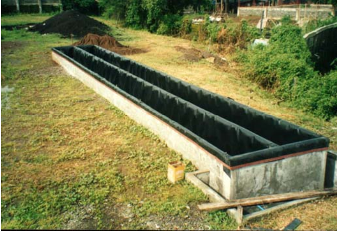
Figure 3-3 The reedbeds after HDPE-liner installation, before placement of soil media.
