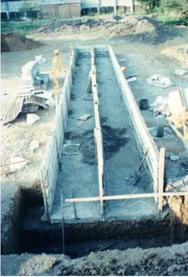
Figure 3-1 Construction of reedbeds, showing elevations of the floor. The outlet zone is in the foreground.
