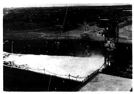
Fig.4 One of the irrigation canal headworks at the Nagarjunasagar Dam on the Kristna River, near Hyderabad, India, for the irrigation of 1½ million hectares (Photo: Douglas Dickins)
