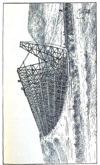
FIG. 32-METHOD OF ELEVATING A HIGH-FLUME TRESTLE.
