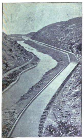
FIG. 33-BENCH FLUME FOR A LARGE CANAL.
