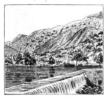
FIG. 20-DIVERTING DAM.
