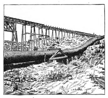
FIG. 28-STAVE PIPE-LINE IN POSITION.
