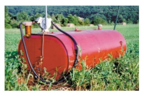
Salvaged 275 gallon horizontal fuel tank with hand fuel pump and filter. This type of pump is suited for all fuels; current use is for diesel fuel..
