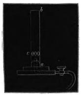
about  $\frac{5}{8}$ ths of an inch in diameter, sliding at a on a fish-tail burner; the air enters by holes at c, the amount being regulated by means of a small slide, which closes them wholly or partially as may be required. The nature of the aperture by which the gas enters is well adapted for causing it to mix with the air, notwithstanding the small size of the tube a b.
